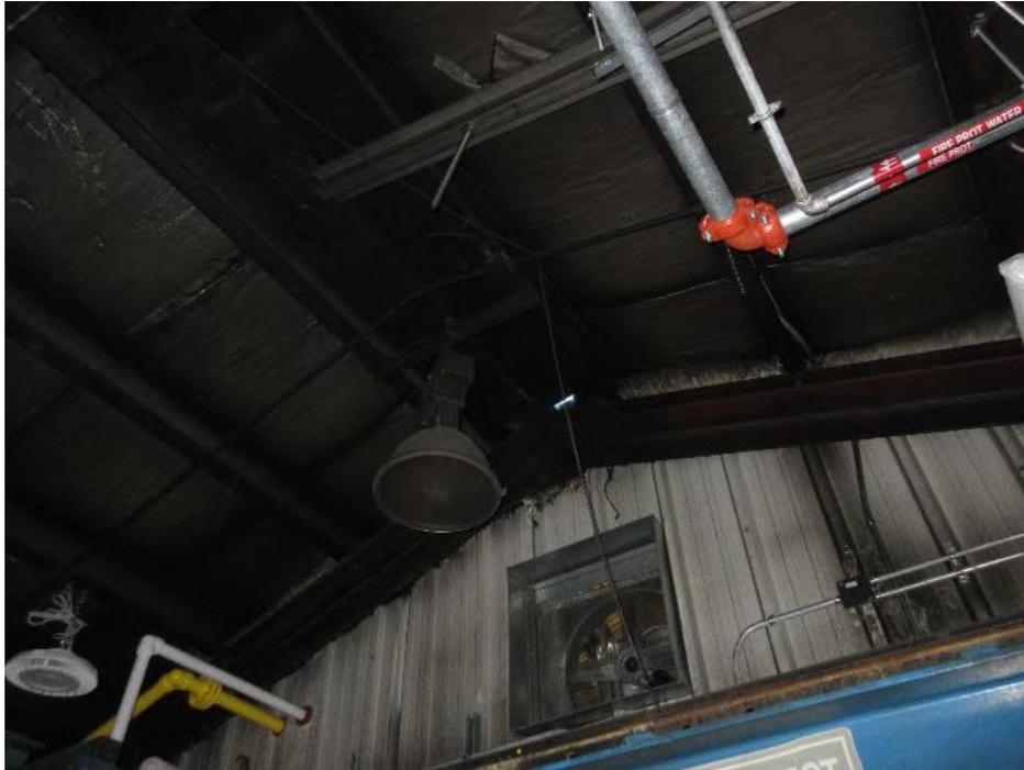
Figure 5: Roof Area where Daylight is Shining Through
