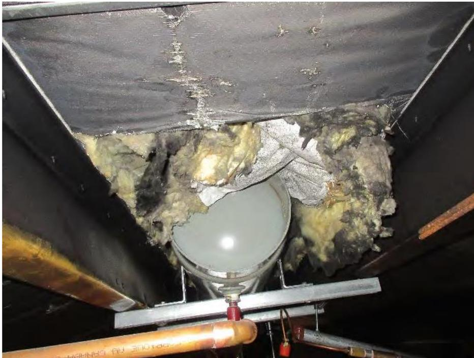
Figure 4: Damage to Interior Insulation of the Building due to Roof Leaks
